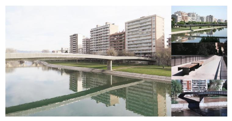
The construction of this pedestrian footbridge over the River Segre in Balaguer has been solved in a most economic and, at the same time, structurally very efficient way. It consists of a pre-stressed beam of two spans of 46,60 m and a T-beam cross section of 5,00 m width, made up of a central rib of 0,50 m width and very slender cantilevers of 2,25 m at each side. The cantilevers that constitute the flanges of the T-beam vary their position in height along the span.
